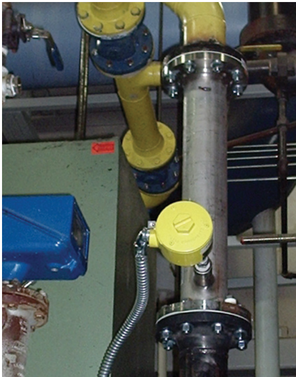
Figure 2: Installed FCI Model ST98 flow meter with Vortab flow conditioner
