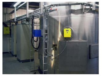
Figure 3. Installed MT91 Flow Meter
