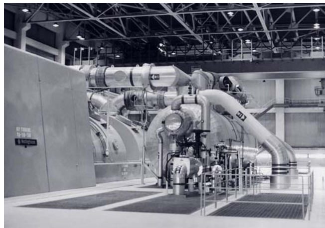
Fig 1. Turbine Air Cooling System
