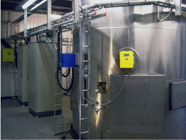
Figure 3. Installed MT91 Flow Meter
