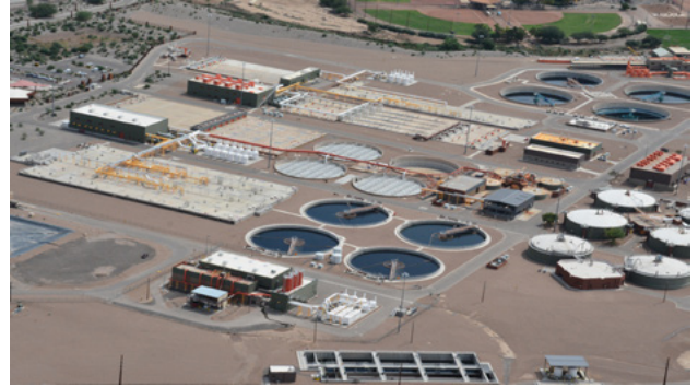
Figure 1: Tres Ríos Water Reclamation Facility
