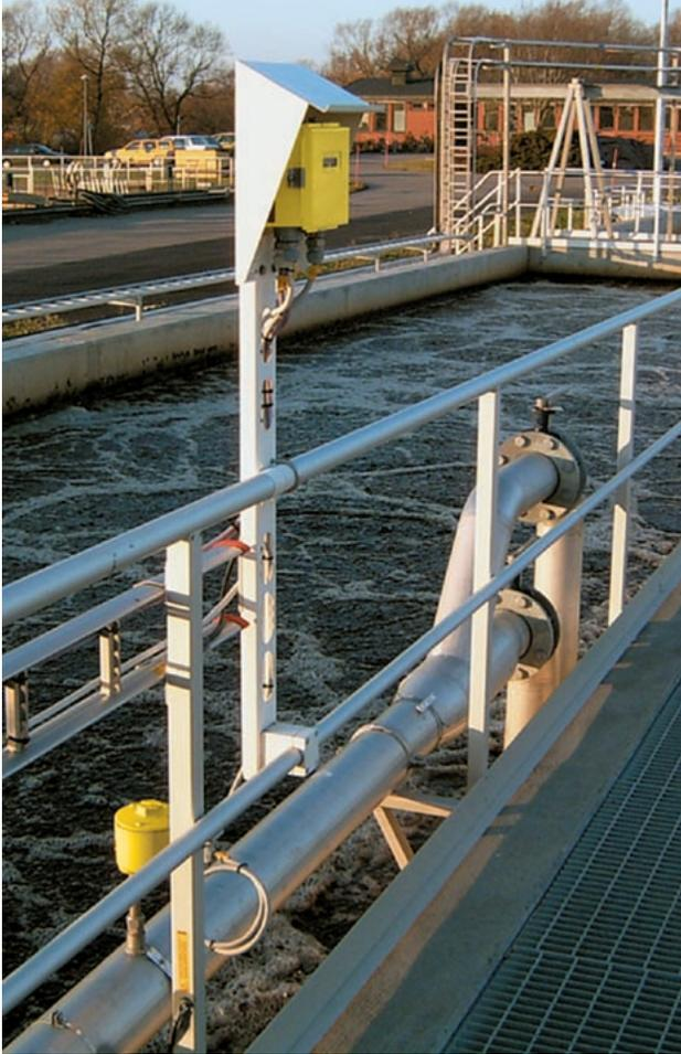
**In municipal and industrial wastewater treatment plants, sludge clarifiers are utilized to separate solids from the water treatment effluent system by introducing air and flocculants. This process results in the sludge rising to the top of the pond or tank and spilling over a weir into a separate collection area. The amount of air and flocculants are controlled by measuring the liquid level interface between the sludge and water.**
