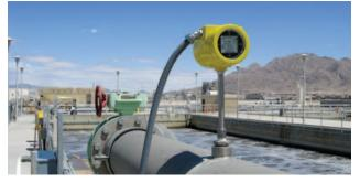
Figure 1. FCI ST100 Thermal Flow Meter at WWT Plant
