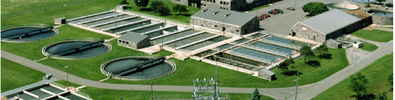
Figure 1: St Cloud wastewater treatment facility
