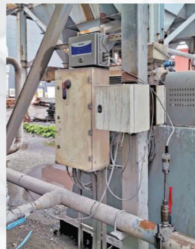
▲ An installed CAL-PM device and FS10i with hot tap installation. Courtesy of FCI
