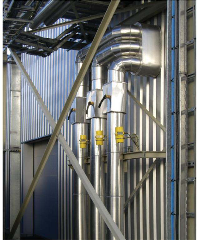
Figure 2. Klargastechnik Equipment With FCI Flow Meters
