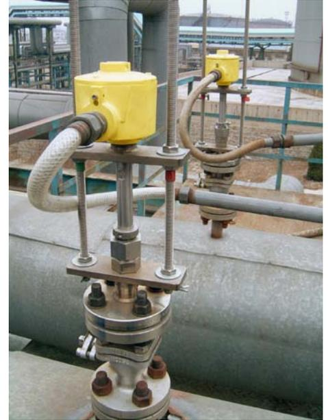
Figure 4: ST110 Flow Meter with packing gland
