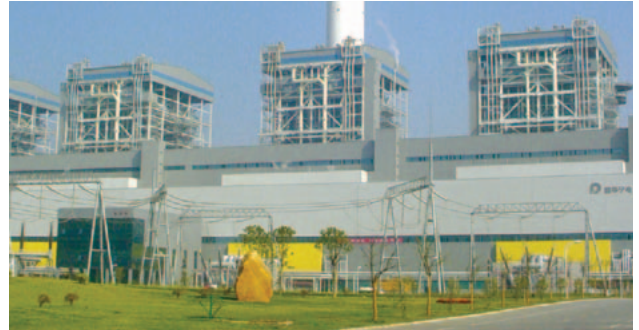
Figure 1: Ninghai Power Plant
